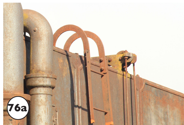
The ladder hooks over the top flange of the tank.
